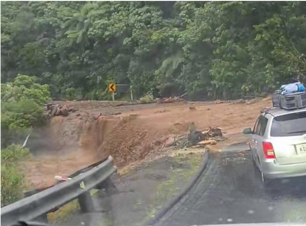
Figure F-3 Floodwater and Debris Encroachment Across Live Traffic Corridor
