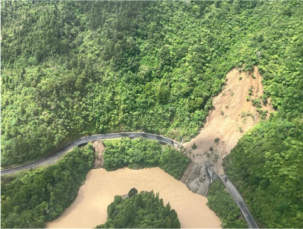
Figure F-2 Major Slip and Hillside Failure Photography
