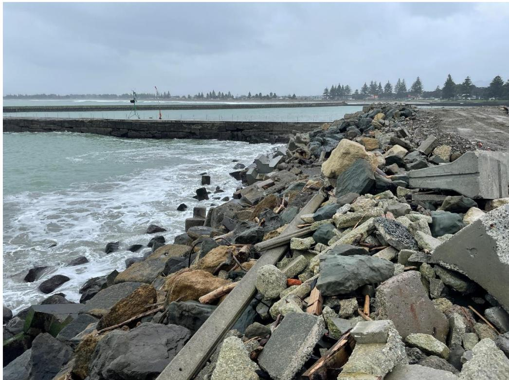
Figure 11: The seawall within the TBP reclamation area is exposed to sea swell and is dominated by large rock spalls and concrete.
