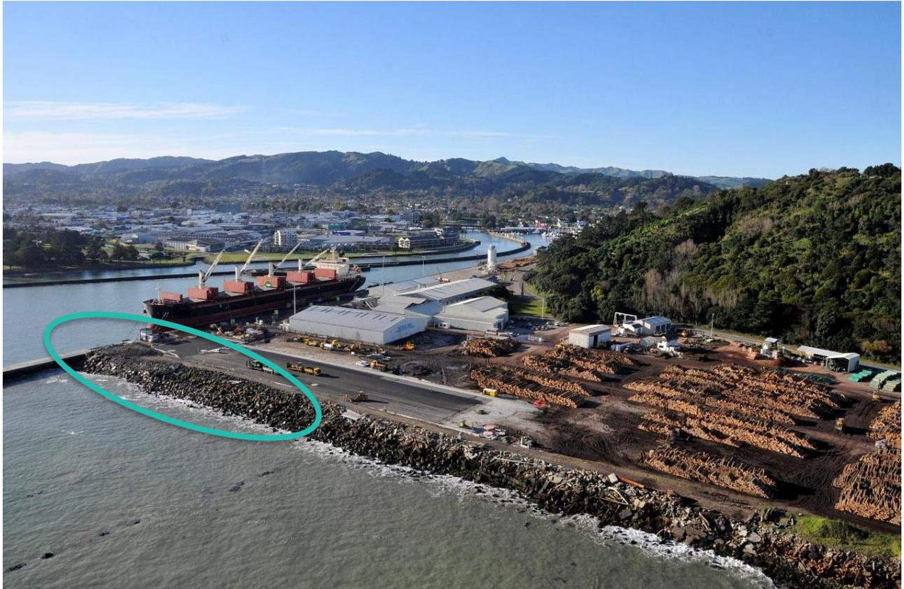
Figure 3: The southern seawall at Eastland Port, looking north towards the Southern Logyard and Gisborne central business district. The area of circled in teal is approximately 130 m of the seawall to be deconstructed as part of the Twin Berths Project (TBP).
