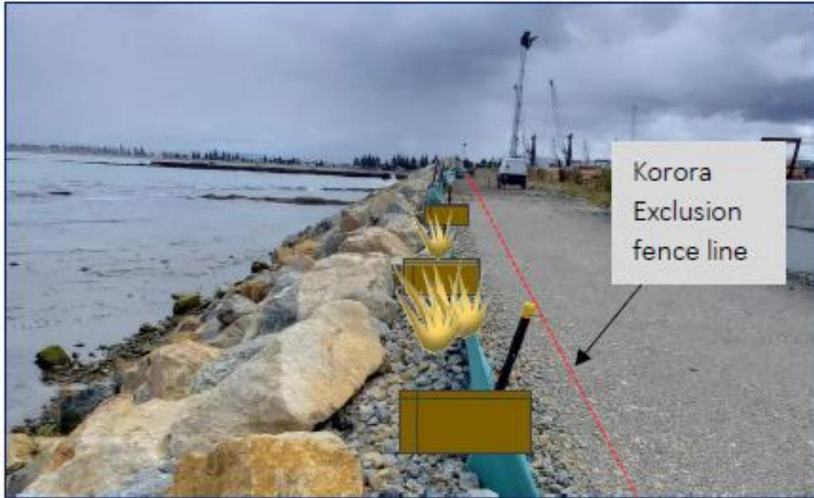
Figure 4: Southern Log Yard Enhancement Area showing indicative nest boxes and Kororā exclusion fence (Source: KCMP Ecoworks 2022).
