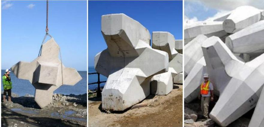
Figure 3-5 – Left – X-bloc® (4 m<sup>3</sup>/9.6 t, Port Oriel, Ireland). Centre – Accropode units (6.2 m<sup>3</sup>/14.9 t, Scarborough UK). Right – Core-loc® (15 m<sup>3</sup>/36 t, Kaunapali Harbor, Hawaii). (Reedjik & Muttray, 2009)
