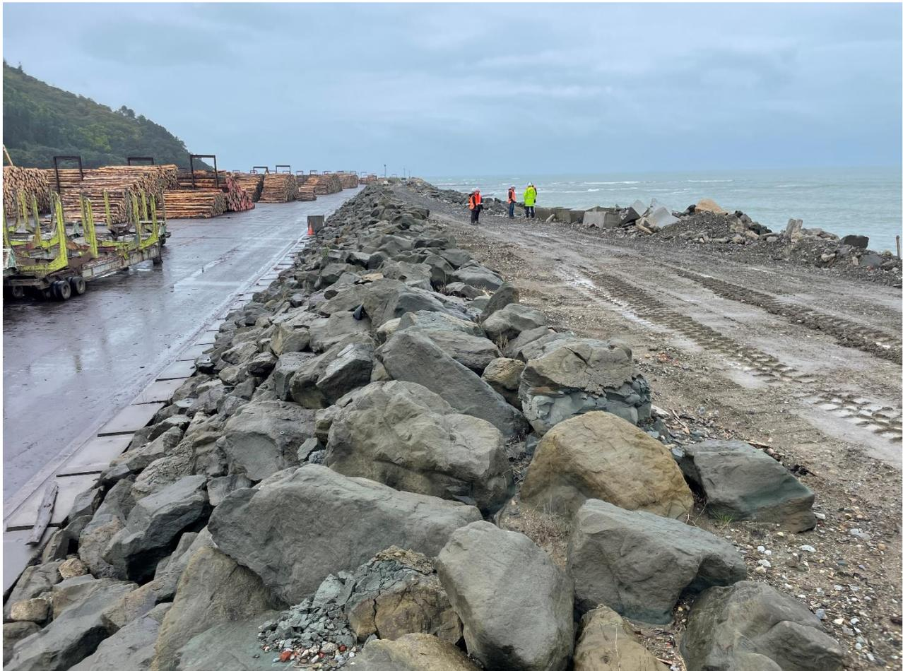
Figure 14: Inner seawall that separates the logyard from the road and the outer seawall.
