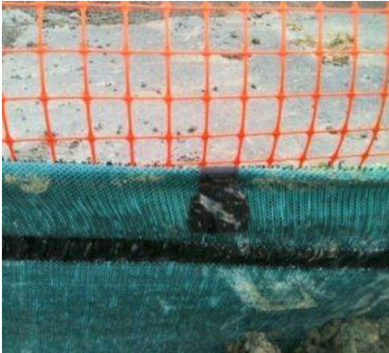
Silt fence correctly secured to the top wire using silt fence clips (Source: Southern Skies).
