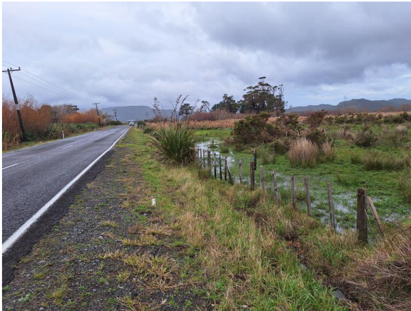
Figure 5. An example of where road safety fencing would be required to be installed within 10 m of a wetland to keep pedestrians safe on the road berm (213 – 214 km).
